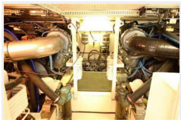
Engine room photo 1
