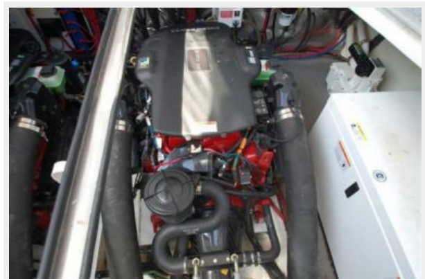
Starboard Engine & Genset
