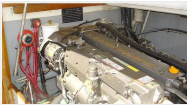
Engine & Mechanical Equipment
